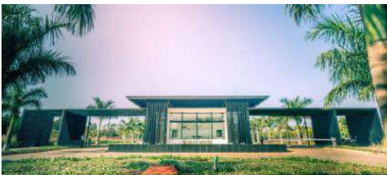
Project visual: Embassy Springs
