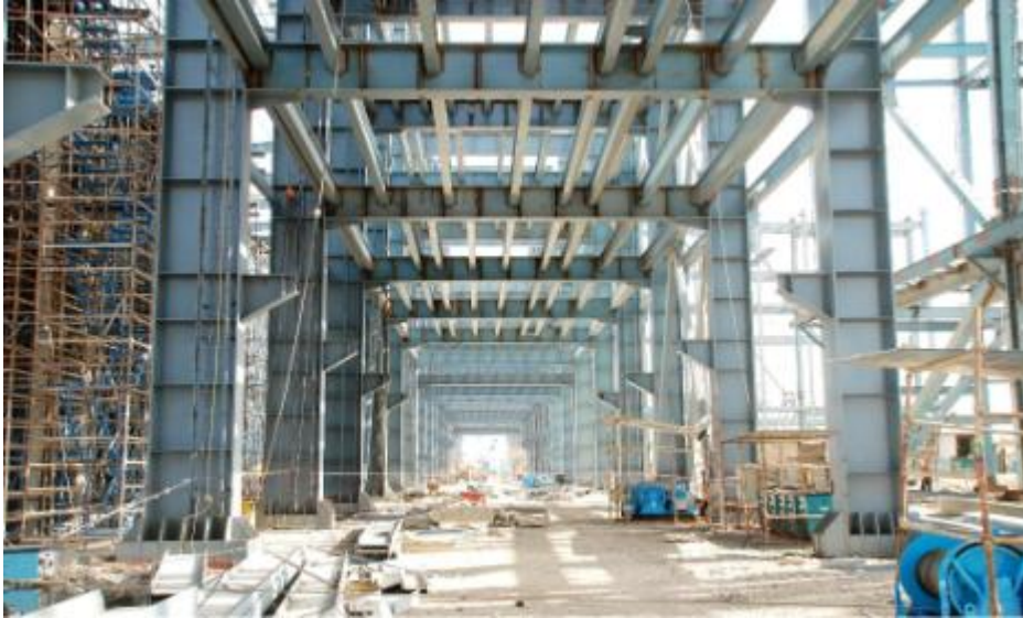
Main Plant Building
