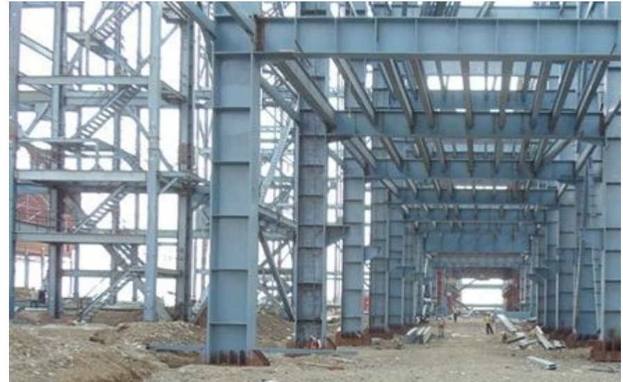
Main Plant Building
