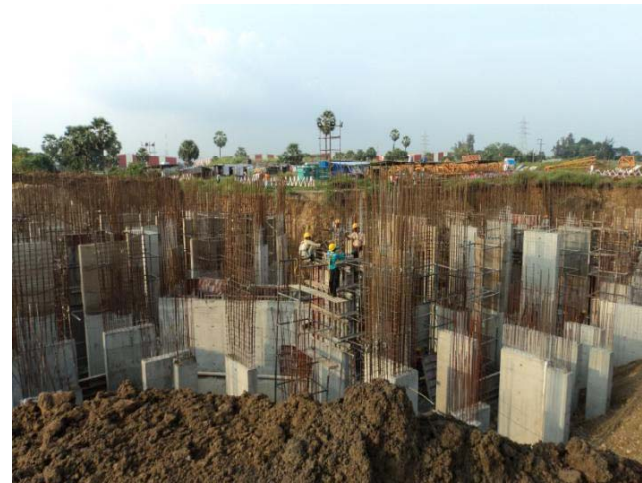
Panvel – Greens work under progress
