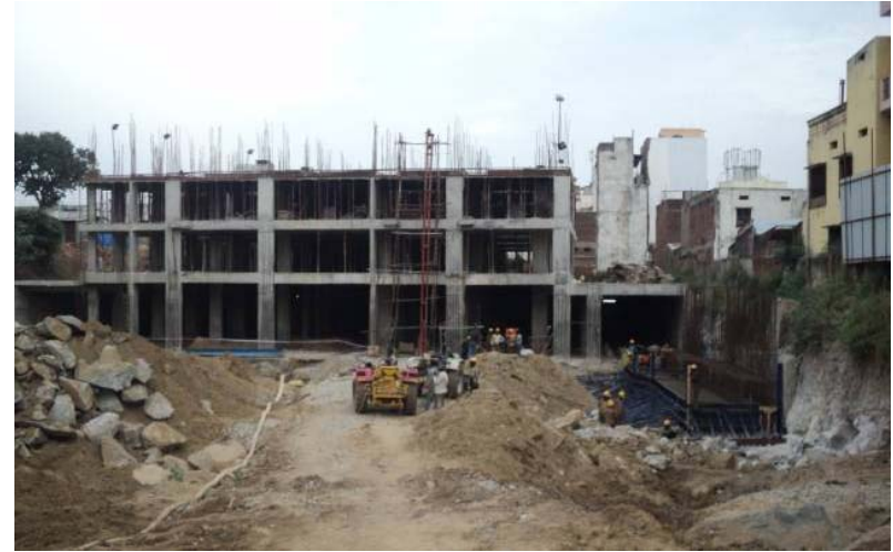
Hyderabad – Central Park Block A 3 rd Floor in progress
