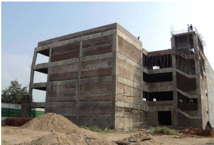
Baroda – High Street Work under progress
