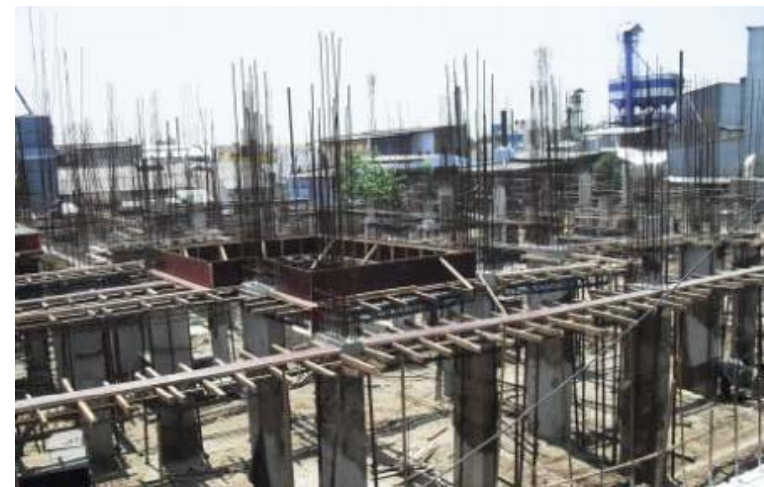
Madurai – Central Park Work under progress
