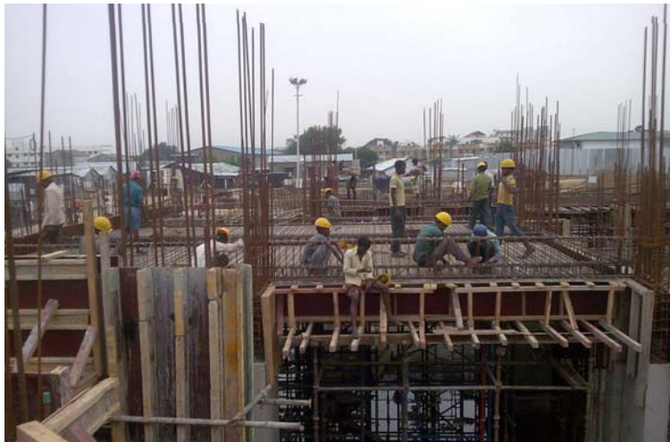
Chennai – Greens Site work under progress
