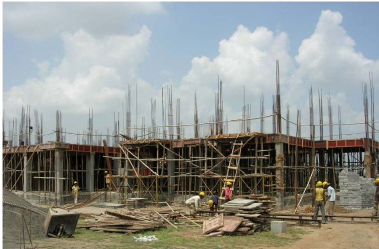
Nashik SEZ work under progress
