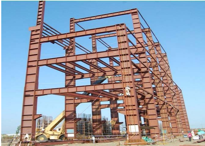
Transformer Generator Building #1
