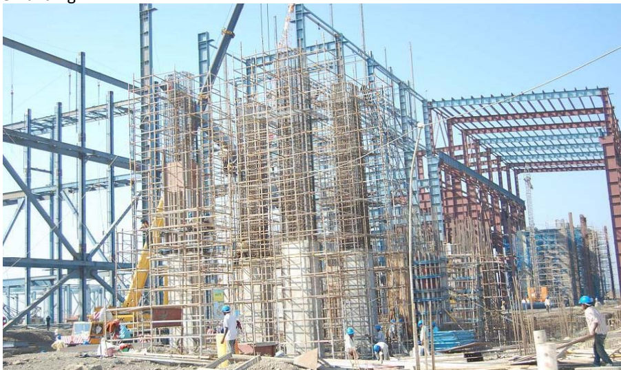
TG Deck Columns
