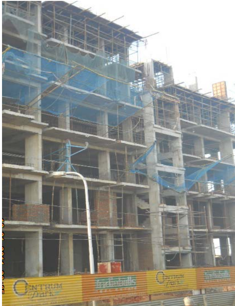
Gurgaon – Centrum Park Project
